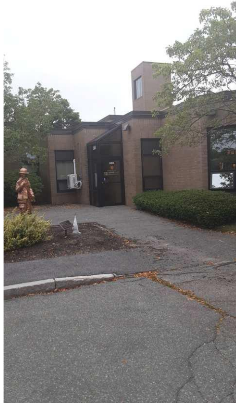
Fire Station 6 West, 540 West Street, Brockton, MA 02301 Inspection Date: June 22, 2023 Inspector: Mark Dempsey
