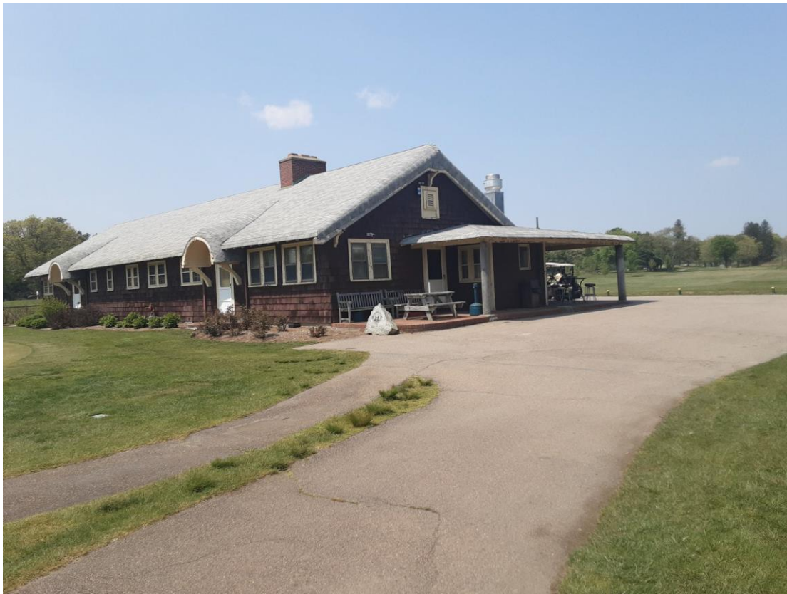
Golf Clubhouse, 331 Oak Street, Brockton, MA 02301 Inspection Date: May 11, 2023 Inspector: Mark Dempsey
