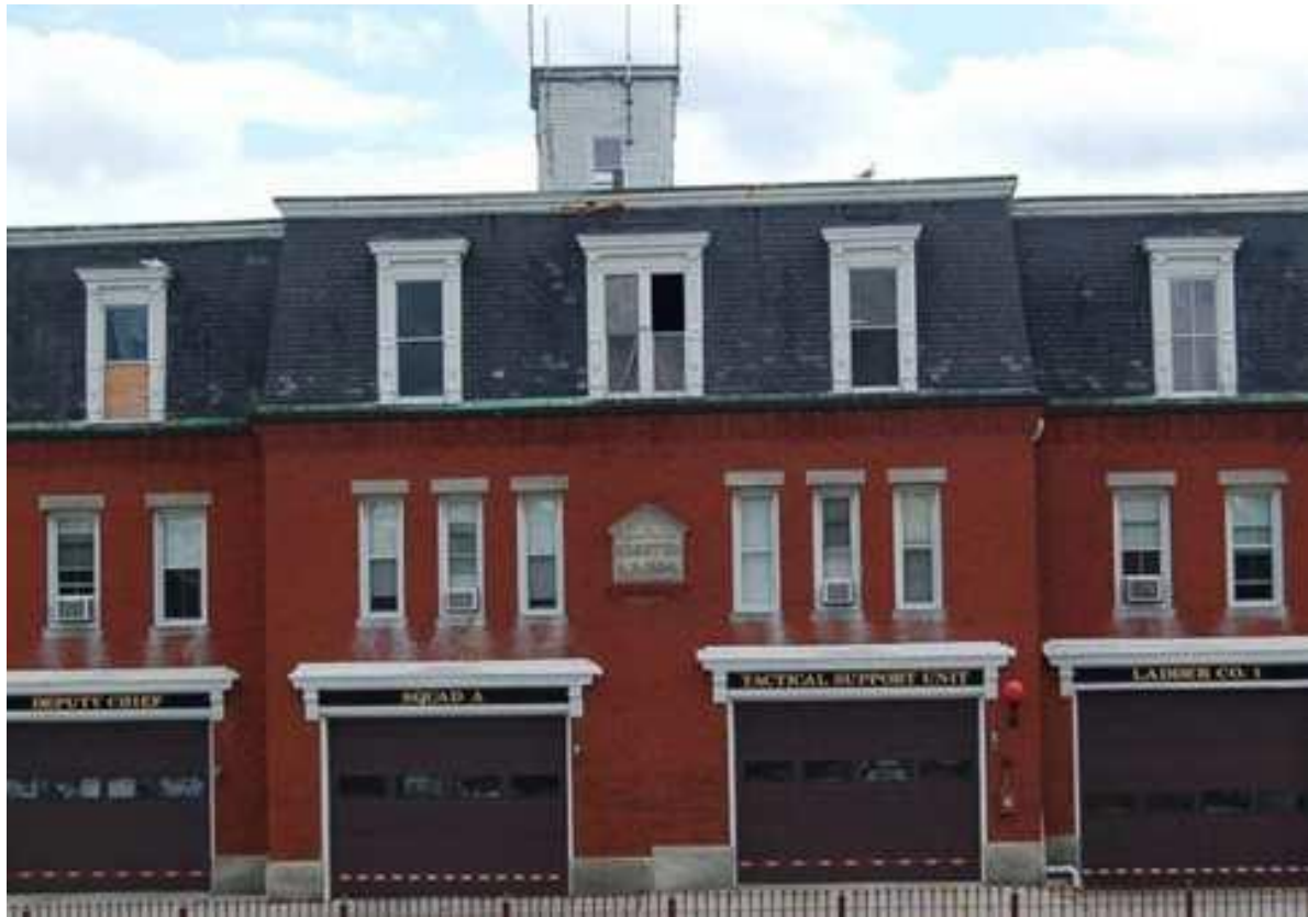
Fire Station 1 Central, 42 Pleasant Street, Brockton, MA 02301
