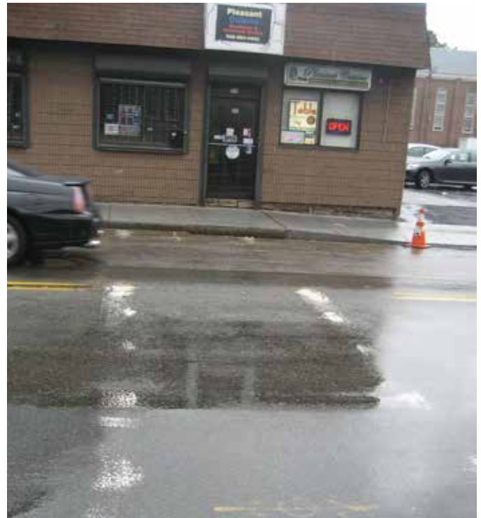
Unprotected mid-block crossing on Pleasant Street
