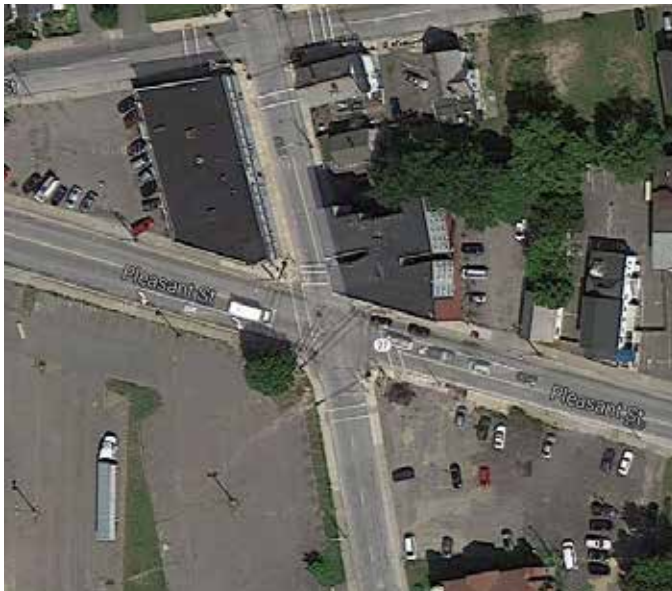
Pleasant Street and Warren Street intersection geometry creates complicated crossing issues
