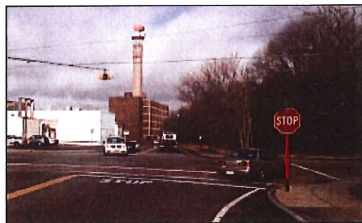
Vegetation to the right of the photo (northeast corner) obscures sight distances for vehicles waiting at stop line on the southbound approach
